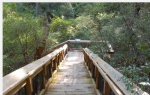
The stairway makes the journey into and out of the crater easy & comfortable.
