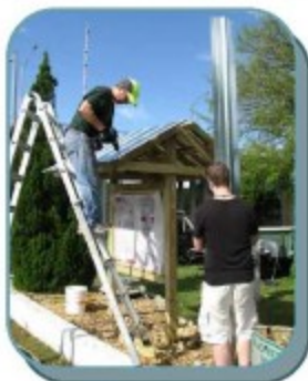
Mike finishing Roof
