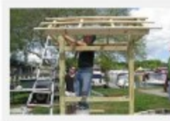
Attaching Roof to Frame
