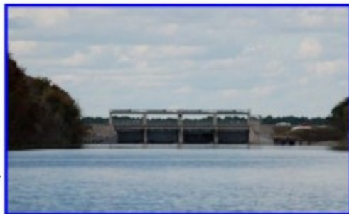
Kirkpatrick (Rodman) Dam located just west of State Road 19, 14 miles south of Palatka.
